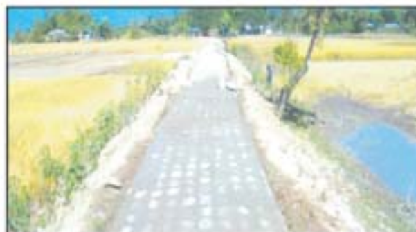
Roads already constructed/under construction with concrete blocks in the Sunamgonj district.
