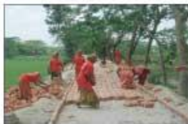
Photograph-66 HBB road being constructed by LCS
