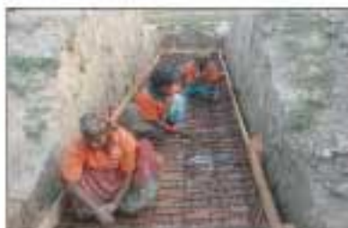
Photograph-65 U-drain being constructed by LCS
