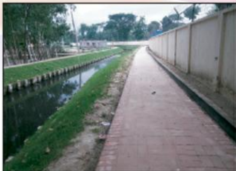
Slope protected along Shama Sundari Canal and footpath constructed alongside.
