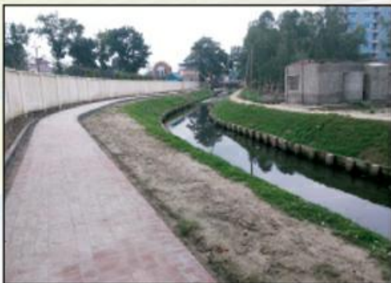
Slope protected along Shama Sundari Canal and footpath constructed alongside.
