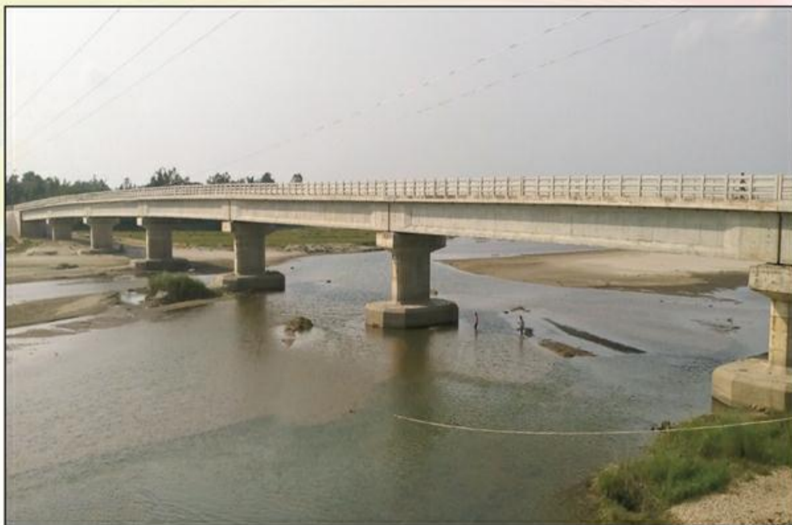
280 meter long PC girder bridge on Kantajir Mandir Road in Dinajpur District .
