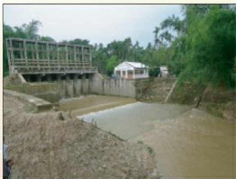
8-vent retention structure at Langulia chara sub-project in Sreemongal under Moulvibazar
