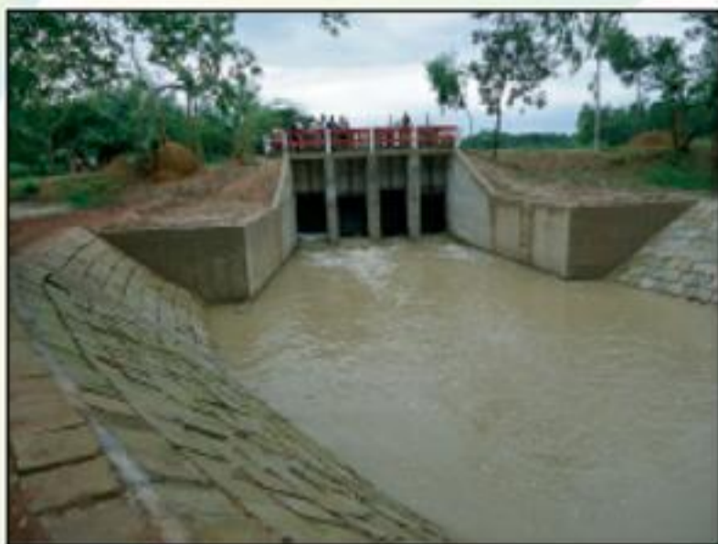
4-vent regulator of salnar canal sub-project in Fulbaria under Mymensingh
