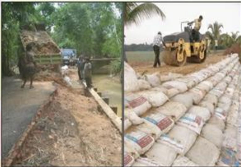
Maintenance work in progress of Chanda-Rajarkul road in Ramu upazila under Cox's Bazar following damage by floods.
