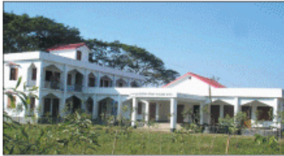
Bulla Union Parishad Complex Building, Habigonj
