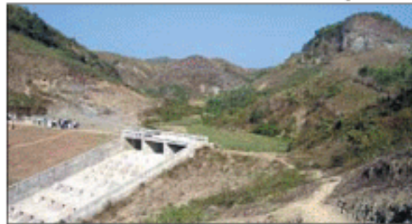
Spillway and reservoir, Shahasradhara Sub-project, Sitakunda, Chittagong
