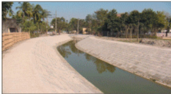
Drain Constructed under Kushtia Pourashava
