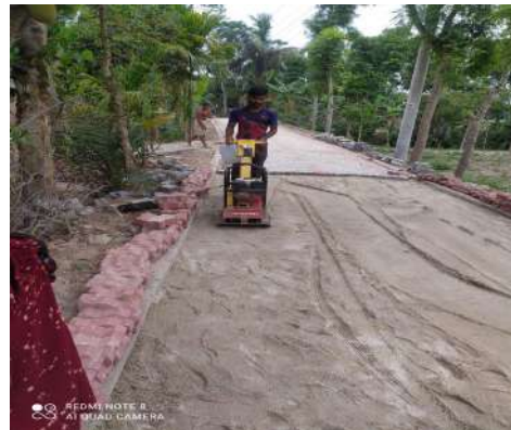
Figure: Compaction of Base
