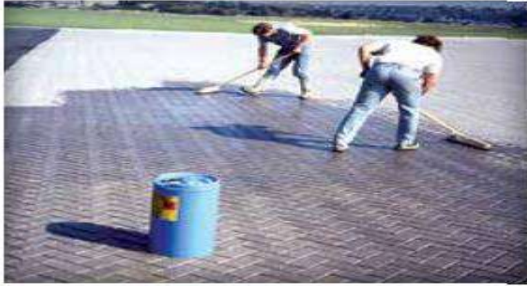
Figure 10. Urethane is applied with squeegees to stabilize joint sand between pavers on aircraft pavement.
