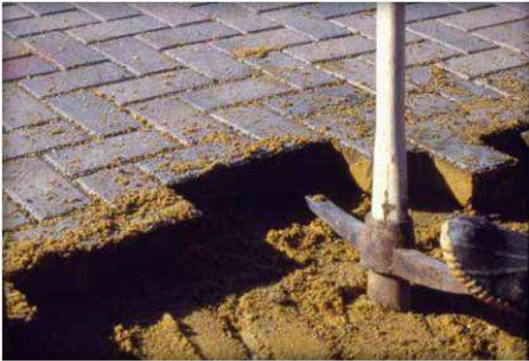
Figure 6. Prying out the remaining pavers
