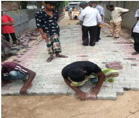
Figure: Block Laying in Stretcher Bond
