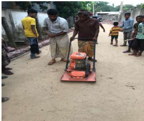
Figure: Compaction of Base
