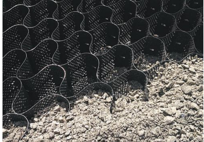
Figure 9. Geocells partly filled with aggregate
