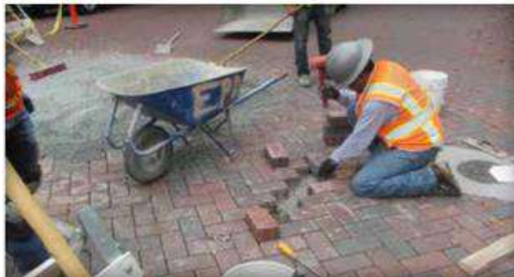
Figure 4. Reinstatement using the same pavers continues following the existing herringbone paving pattern.
