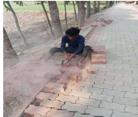
Figure: Cutting and Laying in Stretcher Bond for adjustment with curb stone
