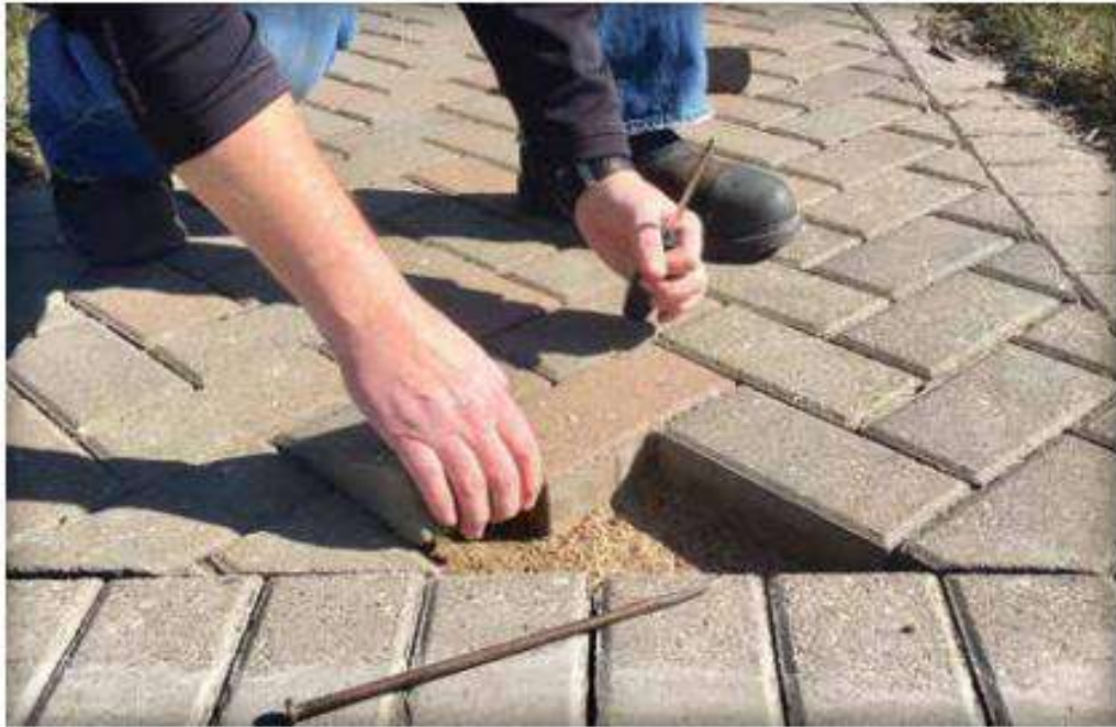
Figure 7. Pulling out a paver by the short end provides greater leverage and makes extraction easier.
