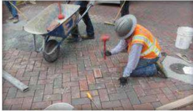
Figure 5. The final paver is inserted, the reinstated area compacted, joints filled, and compacted again. There are not cuts or damage to the pavement surface.
